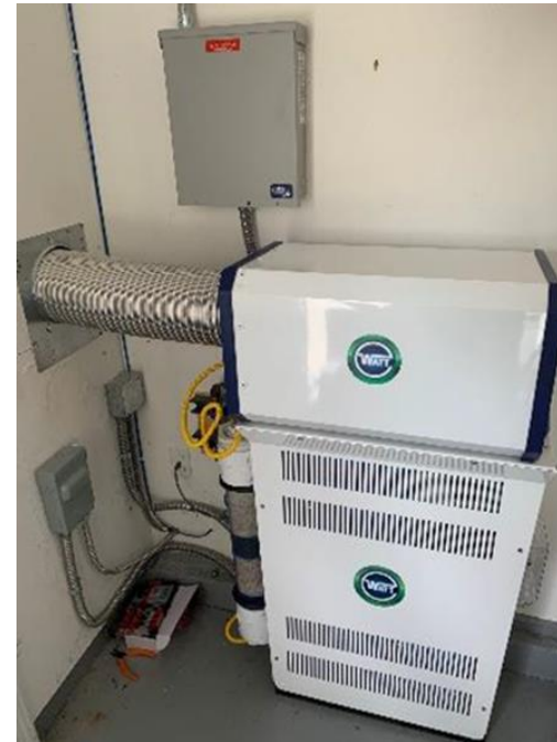
WATT Fuel Cell Home Installation
