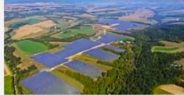
25 MW grid-scale system
